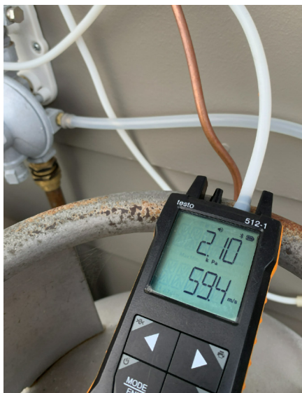
Image shows Integral 2-stage regulator not commissioned, the outlet pressure at the regulator is set at 2.1kPa
