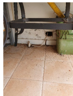
GPO circuit off wall
