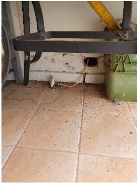
GPO circuit off wall
