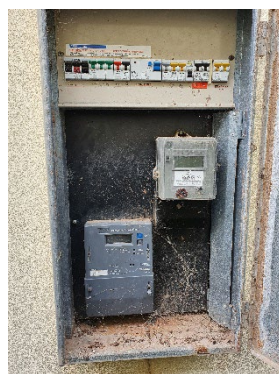
Switchboard Meter Panel
