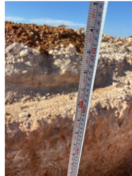
Figure 2 – Investigation hole 1 depth.
