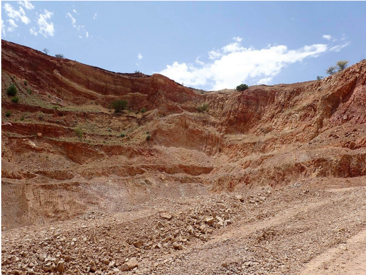
Northern quartzite pit looking south. Minimum floor level is at 183.7 mAHD, 13 m below adjacent drainage line. Floor elevations measured by unmanned aerial vehicle survey (UAV) and accessed via Propeller (2020).
