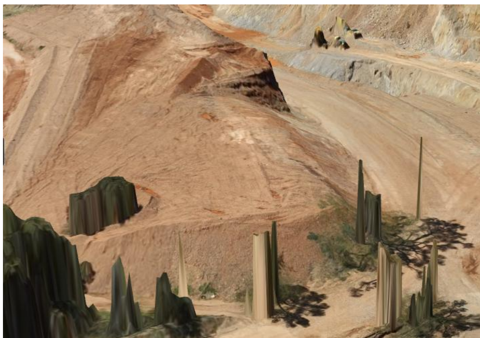
Photo 4 - Battered wall face / rehabilitated area
