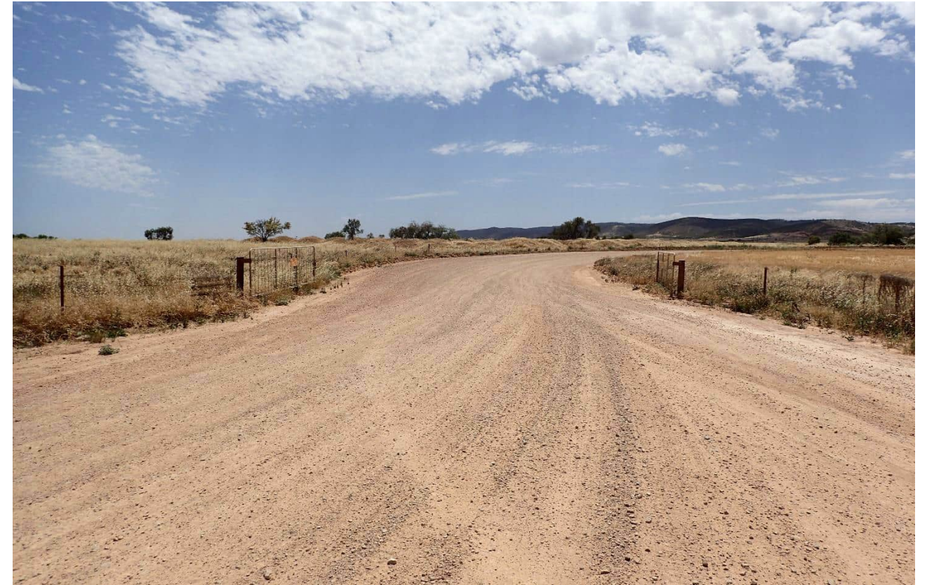
Photo Plate 2: Access road.
