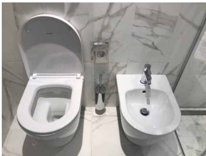
Figure 4: Example of a bidette with an outlet more than 25mm above the rim of the pan.
