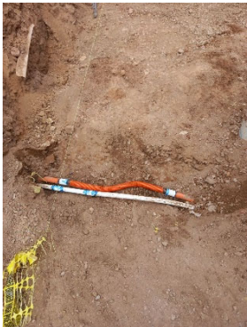
Repaired sub-mains to unit 2
