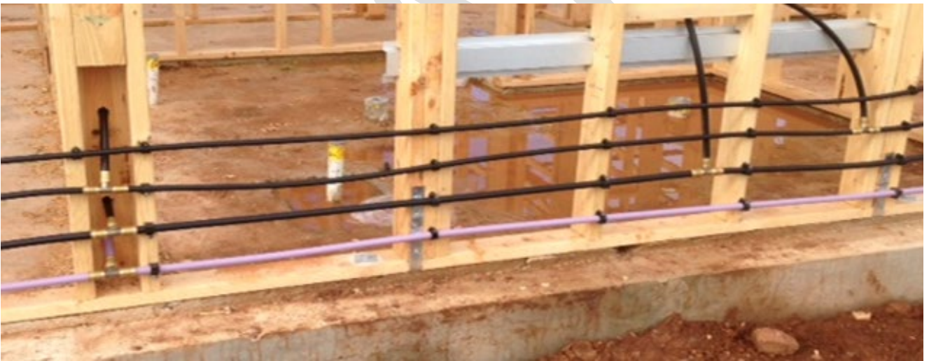
Figure 2-1 In-wall non-drinking and drinking water pipework
