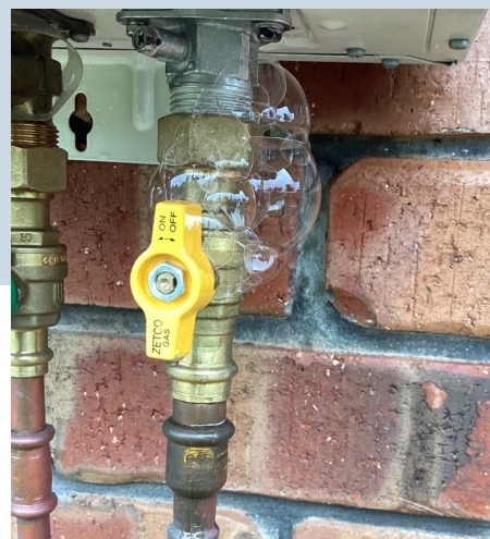
Photos showing different levels of gas leaks at appliance connection points after installation work.
