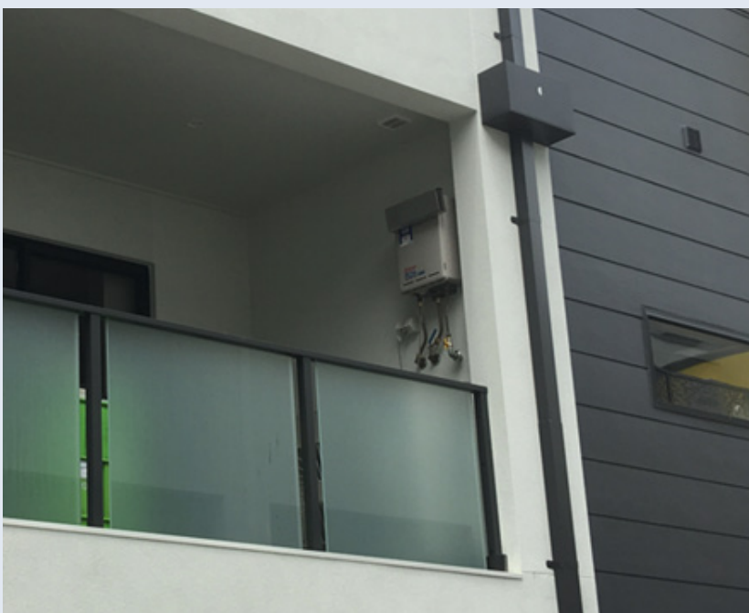
Photo 4: Non-compliant flue terminal location, flue side diverter does not extend past the covered area, the owner could potentially have pull-down blinds installed blocking the flue terminal, creating ventilation hazards.
