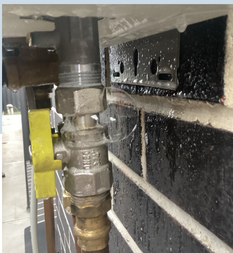
Photos showing different levels of gas leaks at appliance connection points after installation work.
