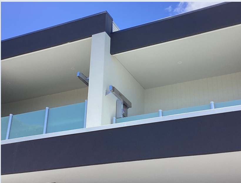
Photo 2: Compliant water heater location with flue side diverters, note flue terminals extending past the covered area.
