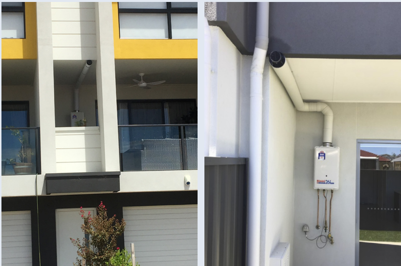
Photo 3: Compliant internal model water heaters installed in an area enclosed on 3 sides under a covered area, note flue kit flue terminals extend past the covered area and down pipe.
