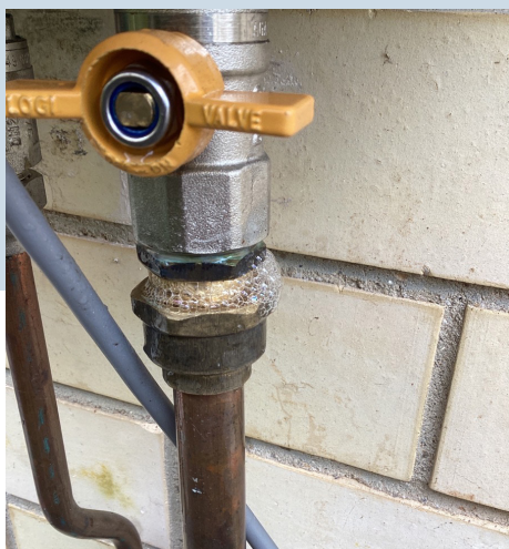
Photos showing different levels of gas leaks at appliance connection points after installation work.
