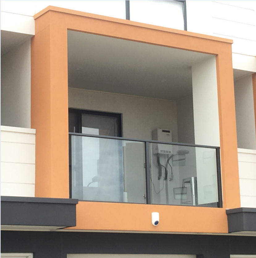
Photo 5: Non-compliant external model water heater installed on a balcony enclosed on 3 sides under a covered area causing a ventilation hazard.
