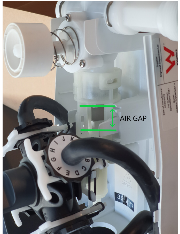
Figure 1 — A chemical dispenser with integral air gap
