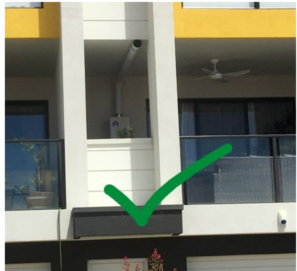
Flue outlet terminating outside opening acceptable
