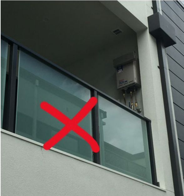
Flue outlet terminating before opening no longer acceptable
