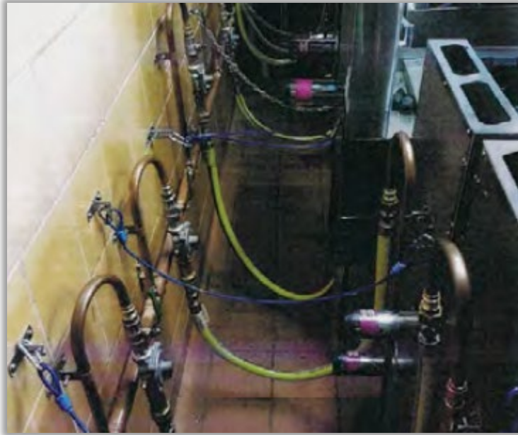
Correct installation method for free standing commercial cooking equipment
