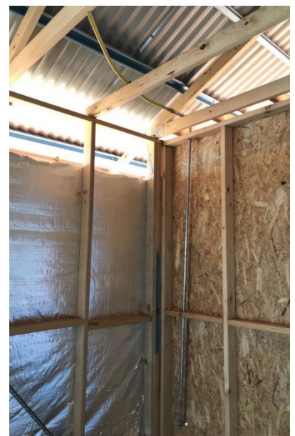
Recommended compliant metallic droppers from the ceiling cavity to the appliance connection points.
