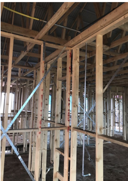
Recommended compliant metallic droppers from the ceiling cavity to the appliance connection points.
