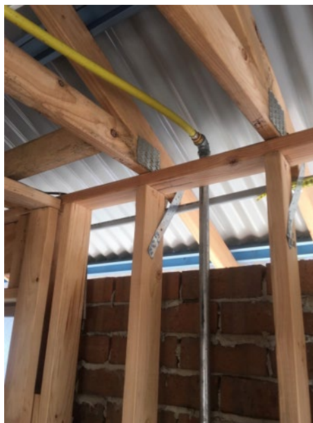
Recommended compliant metallic droppers from the ceiling cavity to the appliance connection points.
