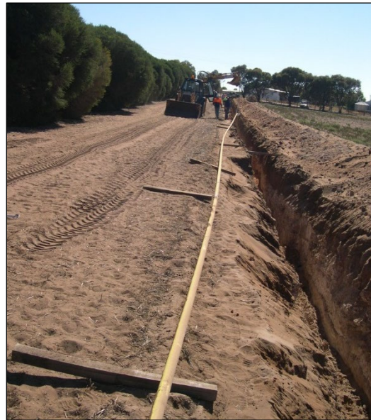
Plate 3-9: Lowering in (Left: large diameter pipeline construction. Right: small lateral construction)
