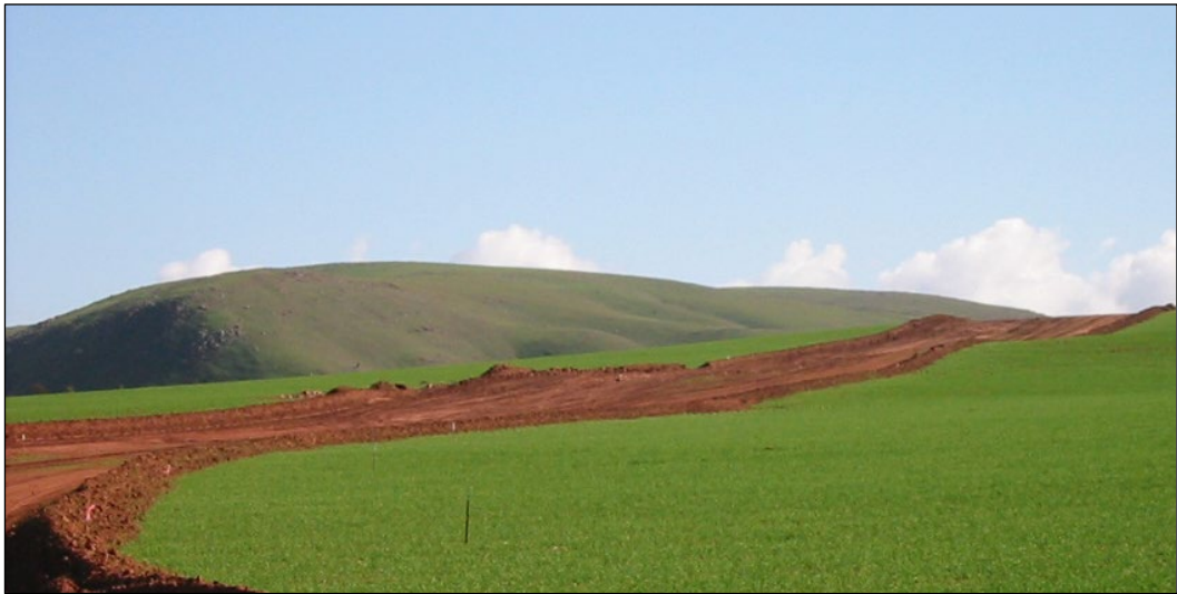
Plate 3-6: Clear and grade (large diameter pipeline)
