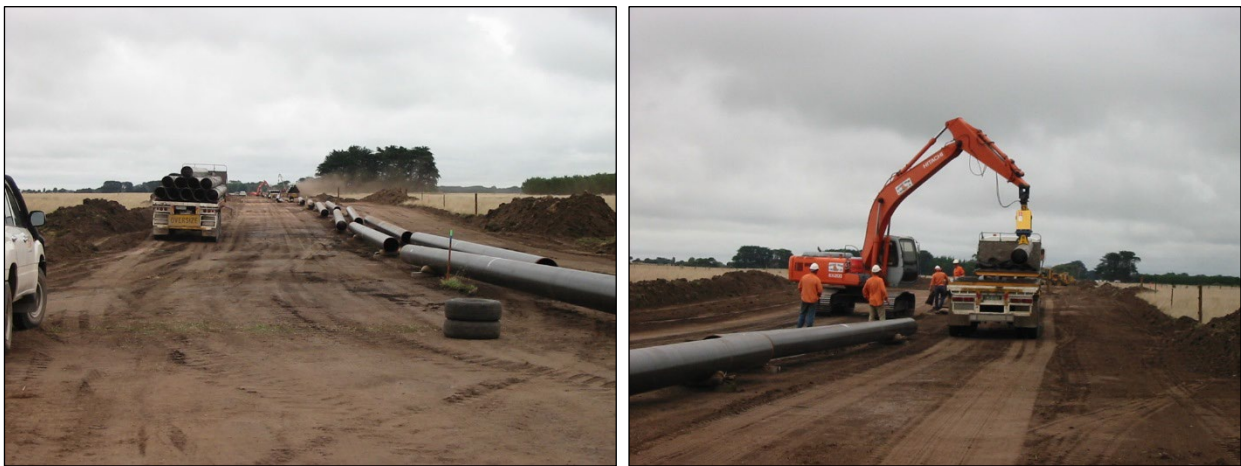
Plate 3-7: Pipeline delivery (left) and stringing (right)
