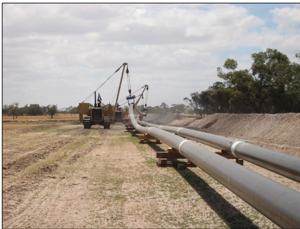
Plate 3-9: Lowering in (Left: large diameter pipeline construction. Right: small lateral construction)
