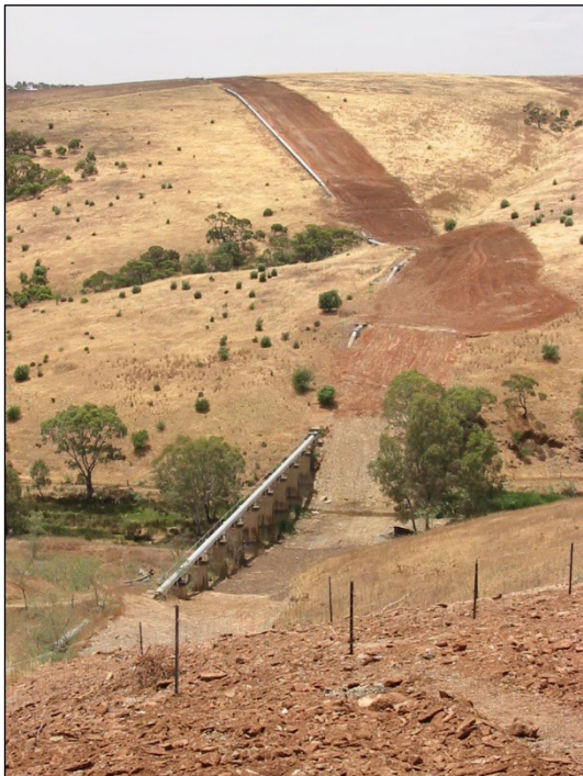
Plate 3-11: Reinstated watercourse crossings (large diameter pipeline). (SEA Gas pipeline is installed on the right of the above-ground water pipeline in the left image)
