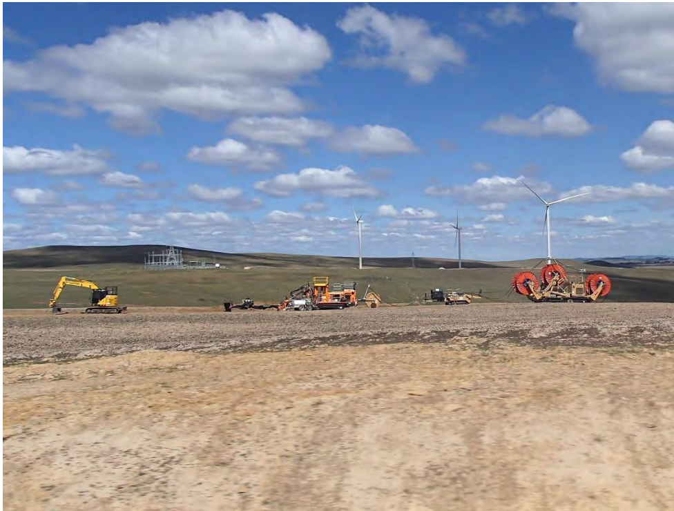
Plate 7 Cable laying equipment (Image: ©GBD 2023)
