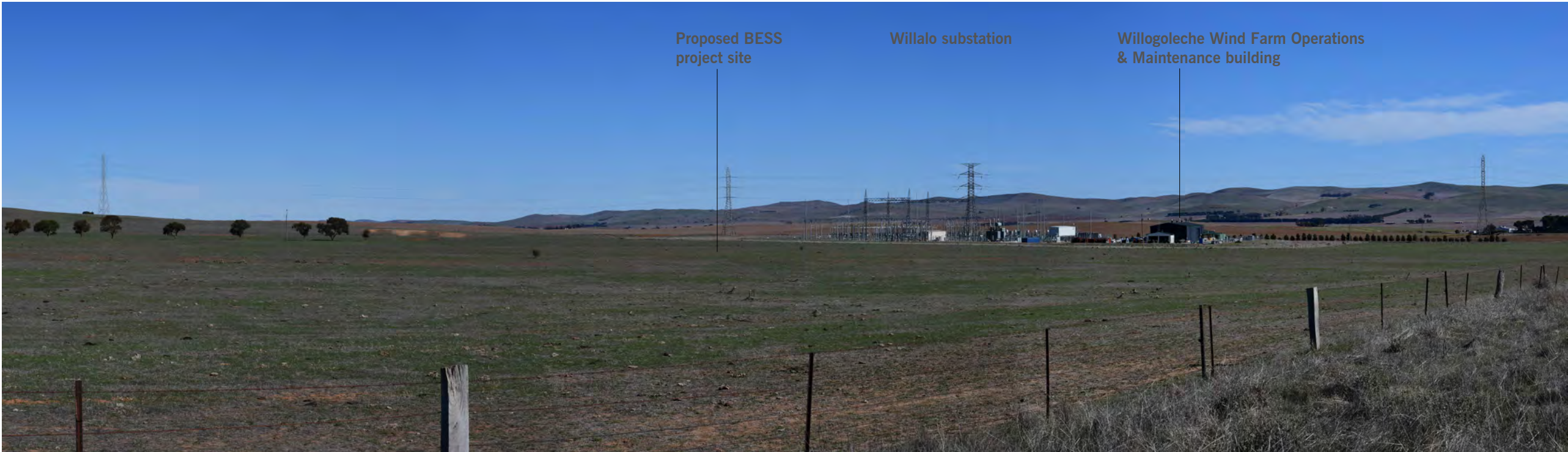
Panorama photo 8 - Existing view south to south west toward the Willalo substation from Willalo Road.
