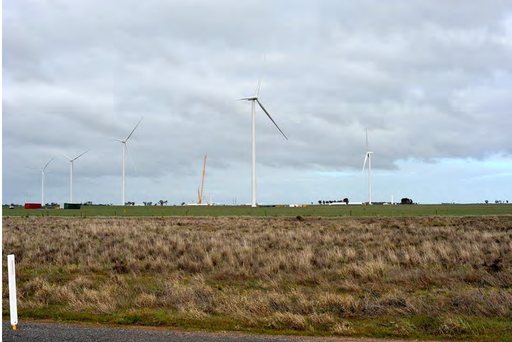
Plate 5 – Typical wind farm under construction (Image: ©GBD 2017)
