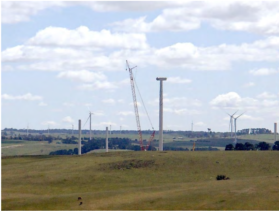
Plate 11 Typical view toward wind turbines under construction (Image: ©GBD 2023)
