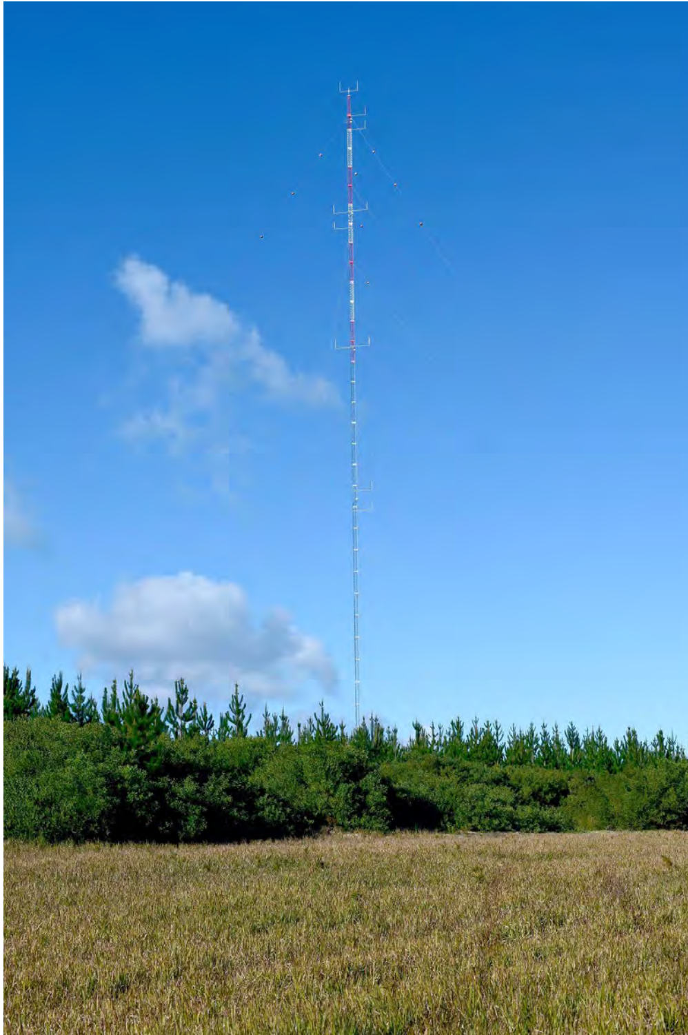
Plate 1 – Typical wind monitoring mast (Image: ©GBD 2021)
