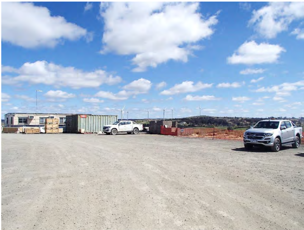
Plate 10 Typical contractors site office and amenities compound (Image: ©GBD 2023)
