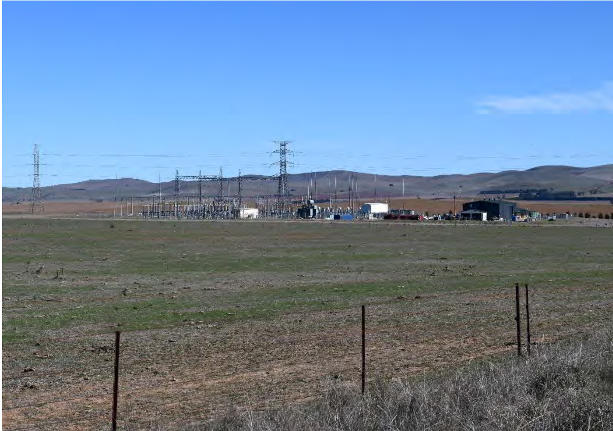
Plate 4 – Willalo substation and operations centre, Willogoleche Wind Farm, Willalo SA (Image: ©GBD 2024)
