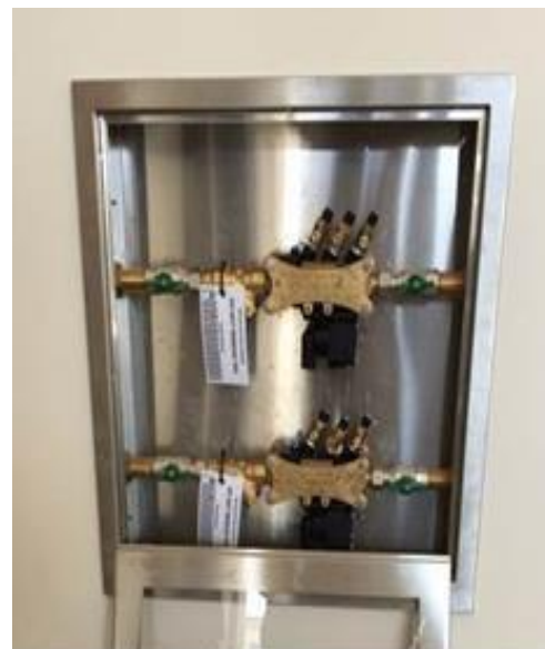
Figure W 15: Reduced Pressure Zone Backflow Devices in in-wall stainless steel tundish box
