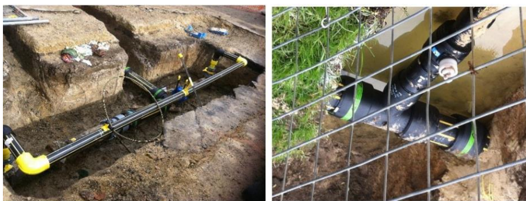
Figure G 3: HDPE mains replacement
