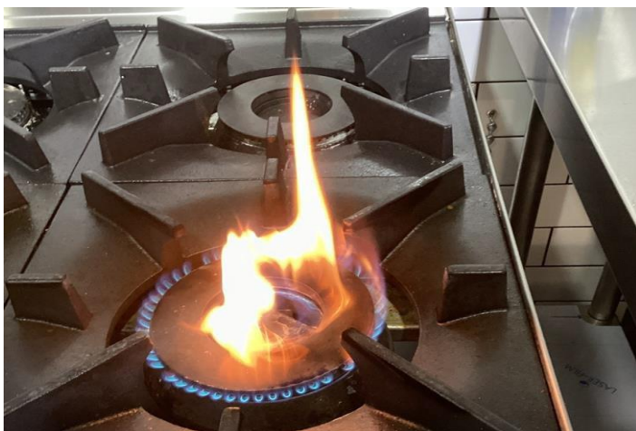
Figure A1 G 16: Non-compliant installation appliance not commissioned
