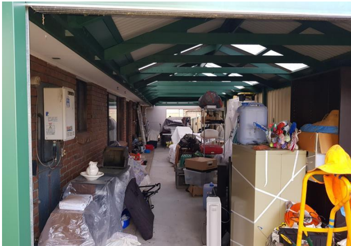
Figure A1 G 15: Non-compliant HWS location
