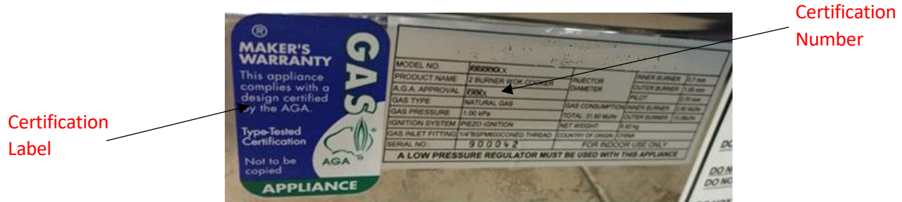
Figure G 16: Information Data Plate including certification number and certification label
