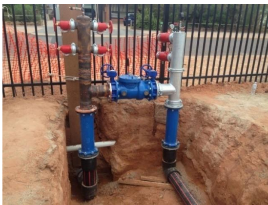
Figure W 13: Fire Service Installation with Backflow Prevention Device
