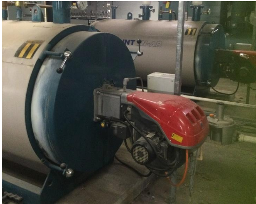
Figure A1 G 12: Photo of a Type B steam boiler
