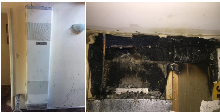
Figure G 13: House fire because of an incorrect DIY appliance installation
