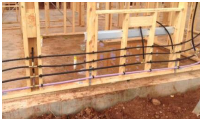
Figure W 12: Plumbing installation showing in-wall non-drinking and drinking water pipework
