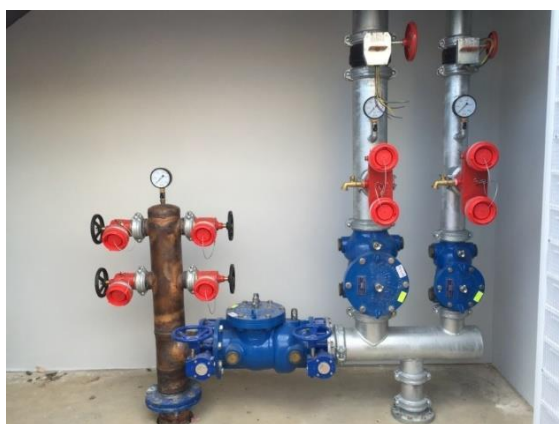
Figure W 14: Variation to a standard fire hydrant booster service
