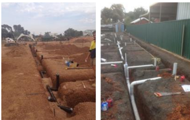
Figure W 4: Examples of Plumbing and Drainage Installations in residential developments
