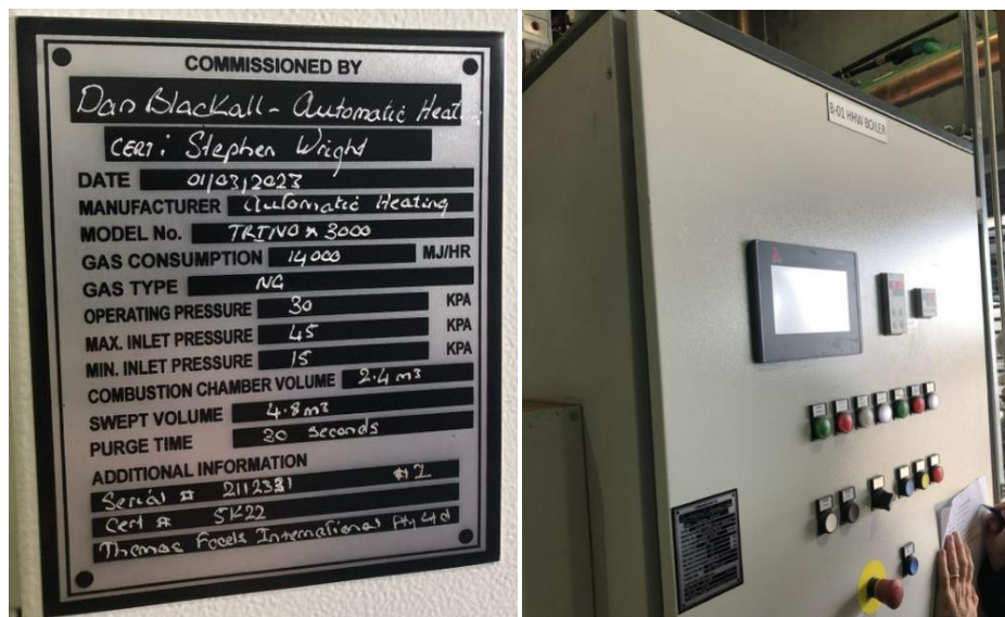
Figure A1 G 13: Typical Type B appliance certification badge plate affixed adjacent to appliance controls.
