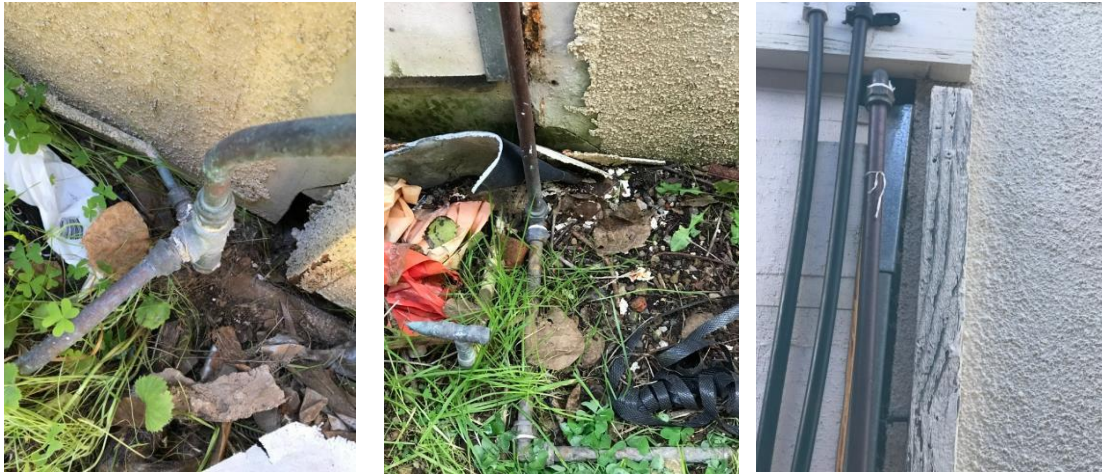
Figure A1 G 14: Failed outlet service
