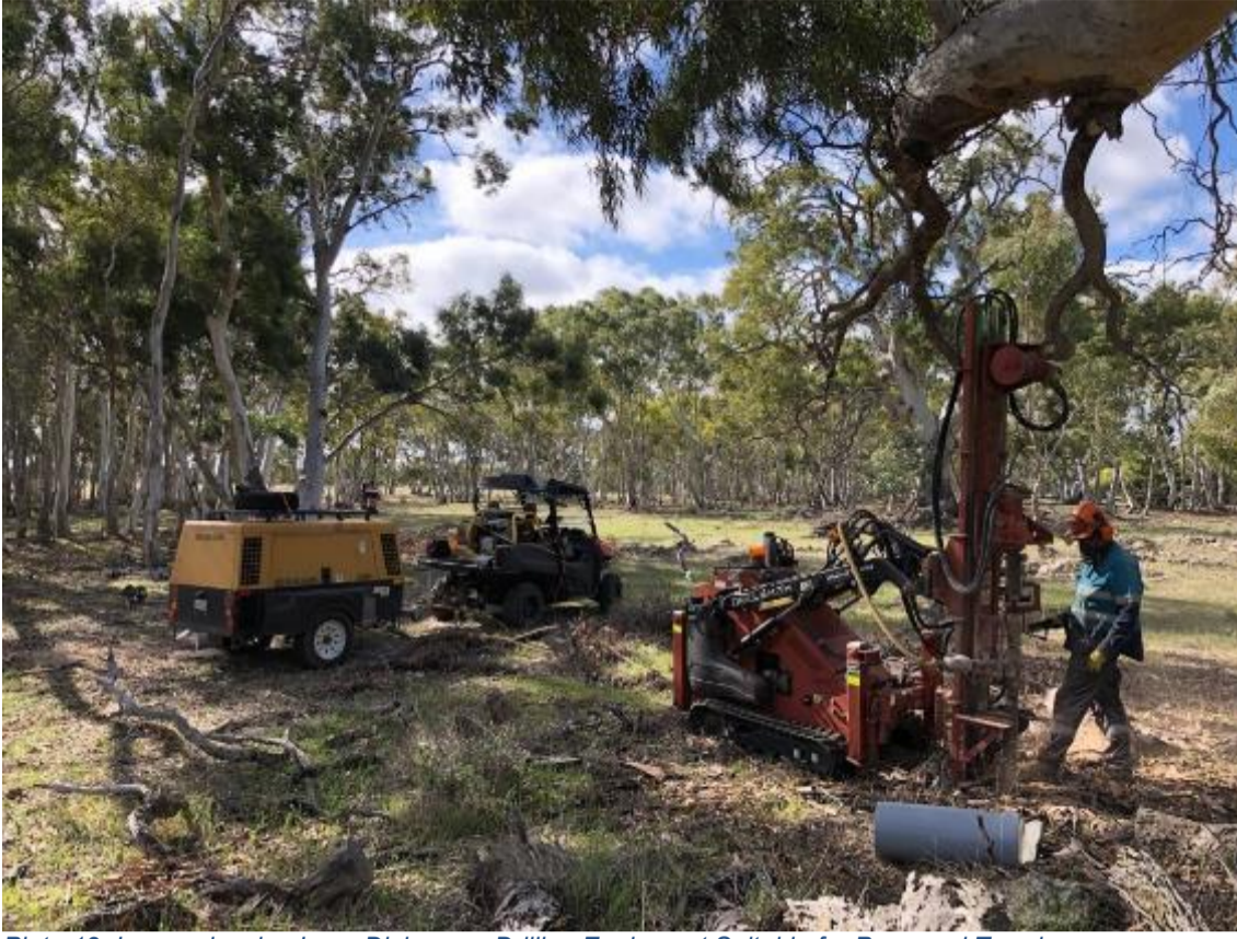
Plate 12: Image showing Leon Dickenson Drilling Equipment Suitable for Proposed Terrain
