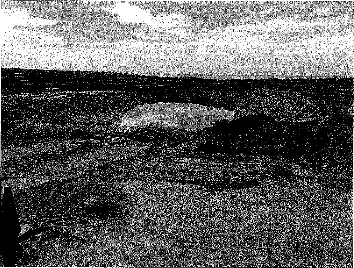
5) Hillside drill tailings dam. Note the gully & gulf in the back ground.
