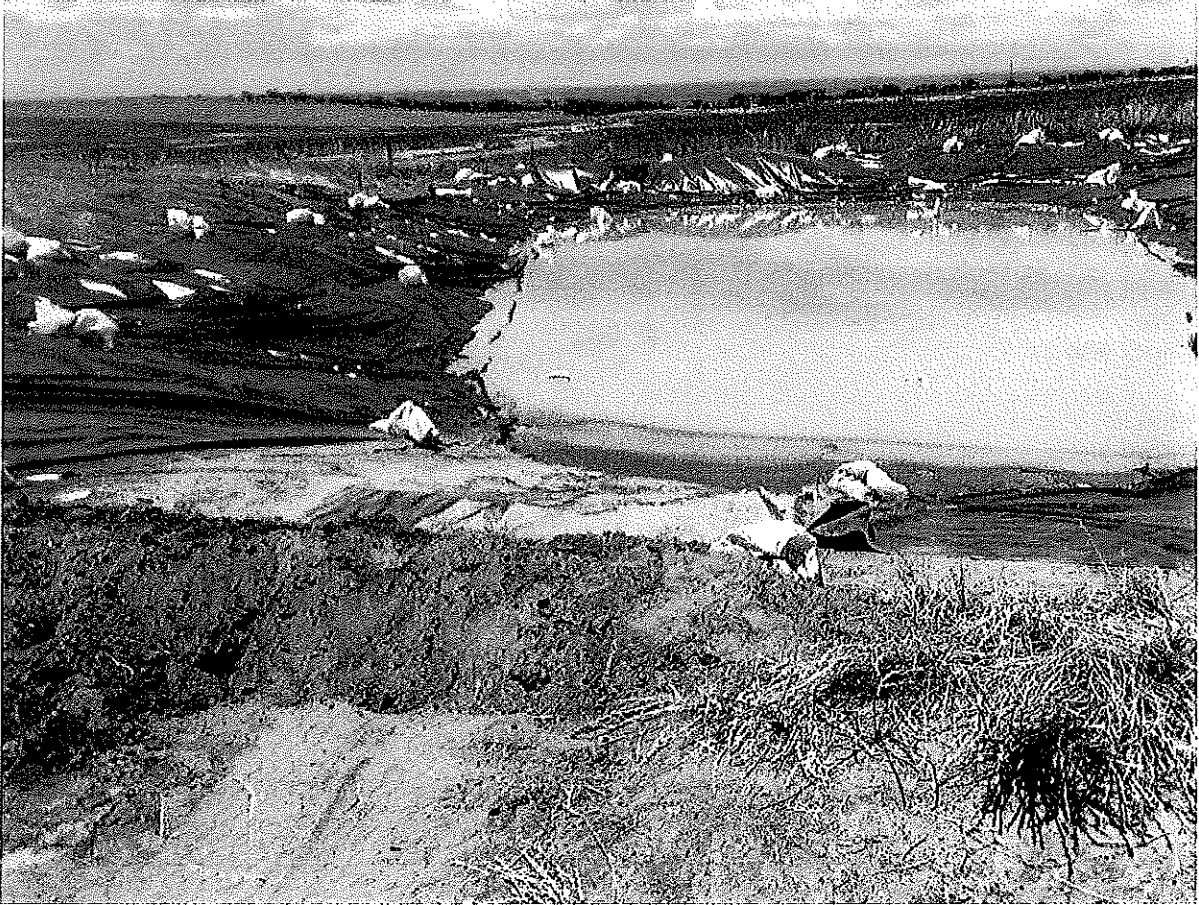
3) Makeshift drill tailing dams with gully & gulf behind.
