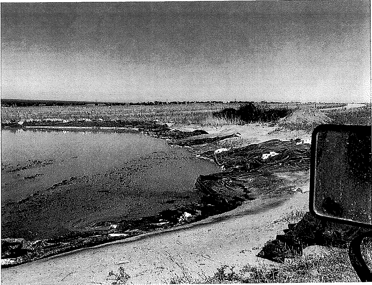
4) Hillside Tailings dam
