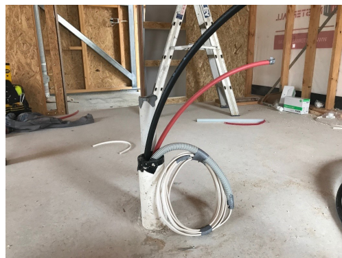
Figure 2 - Non-compliant installation (electrical cable in sleeve with water pipes)
