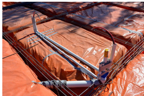
Figure 1 - Acceptable island bench installation using sleeve
