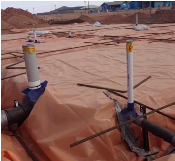
Figure 1: U-PVC pipework installation crossing concrete footing. This installation includes pipe support in the form of a bracket and support.
