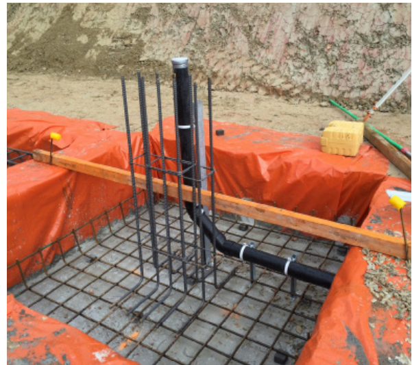
Figure 2: HDPE pipework installation professionally engineered to be installed in concrete structure. The installation includes brackets and support.
