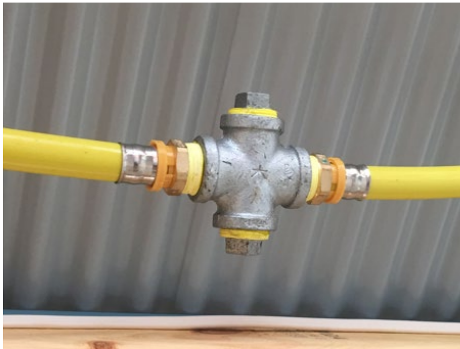
Figure 3: Reversion to BSPT Malleable C.I Cross Fitting - acceptable in South Australia
