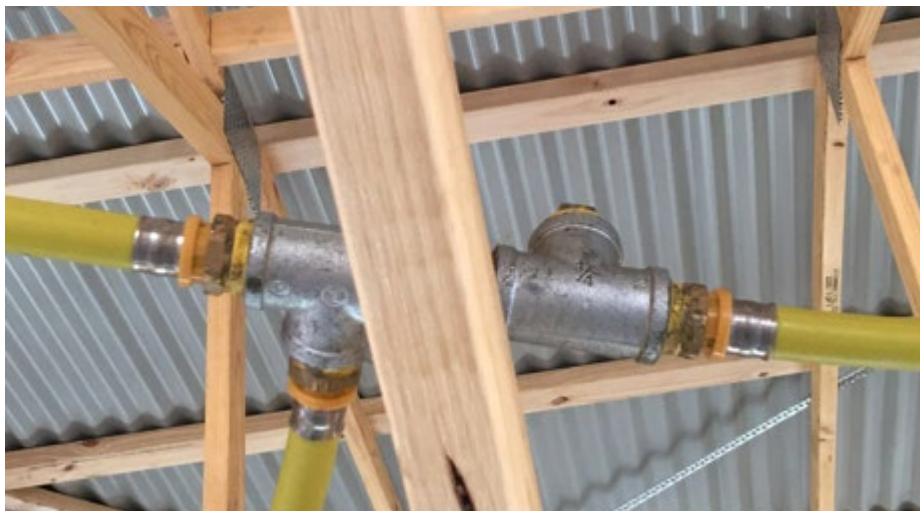
Figure 4: Reversion to 2 joined BSPT MI tees - acceptable in South Australia
