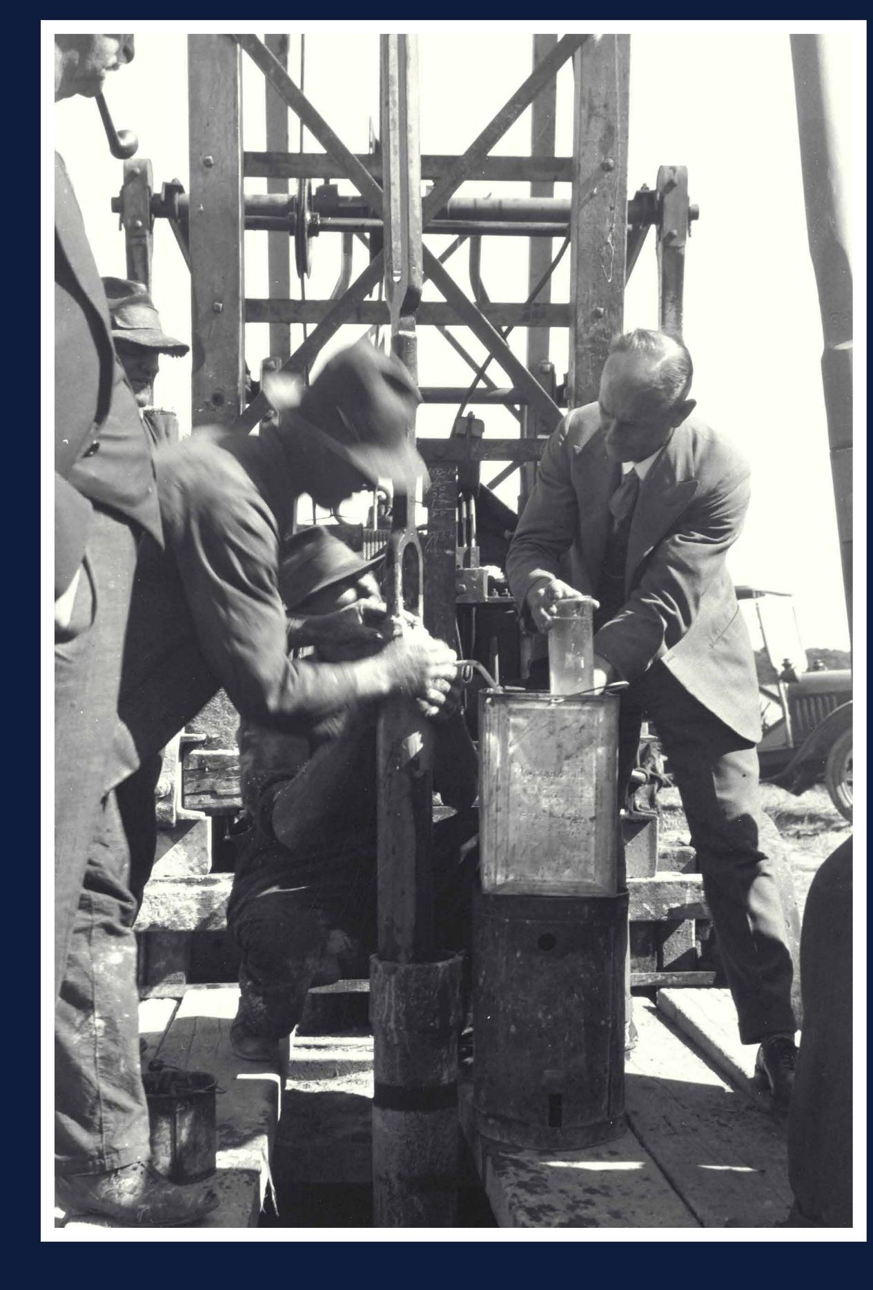
3. Collecting gas from the Ramsay Oil Bore 1 near Minlaton in 1931. The well reached ~548m, and a small gas flow of almost pure hydrogen was recorded (SADEM photograph
