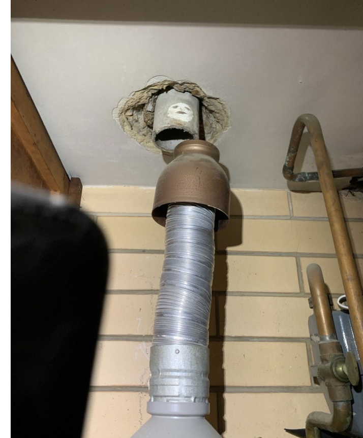
Clause 6.7.4 requires all flue gases to be exhausted to the outside atmosphere
