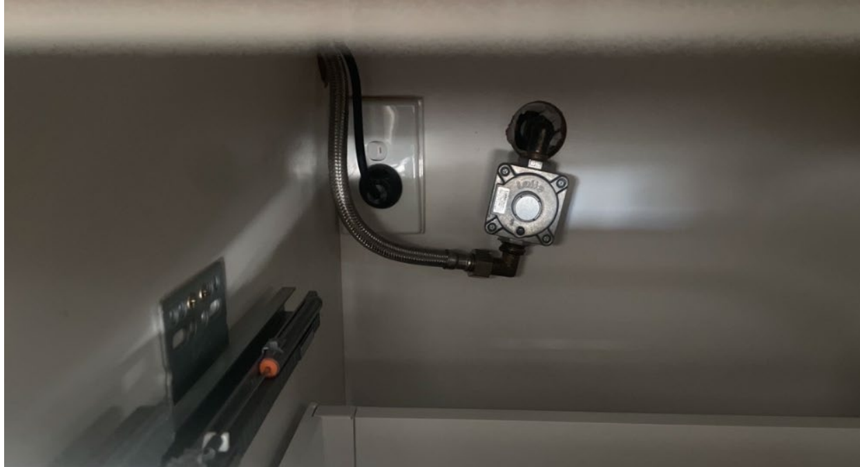
Clause 5.9.6 requires a manual isolation valve and a union fitted at the inlet end of the hose assembly
