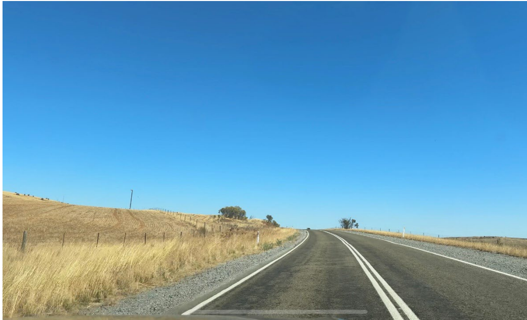
Figure 7 - Crest and curve in Wilkins Highway to the north-west of Weirs Gap Road
