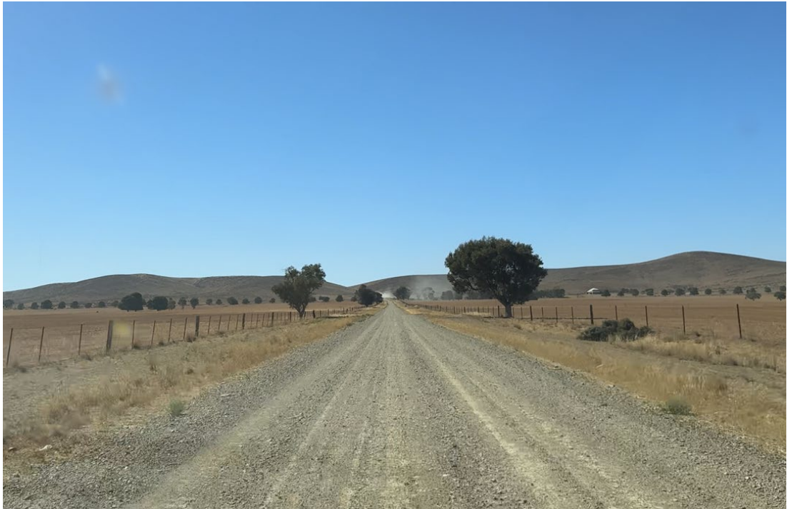
Figure 5 - Weirs Gap Road (looking east)
