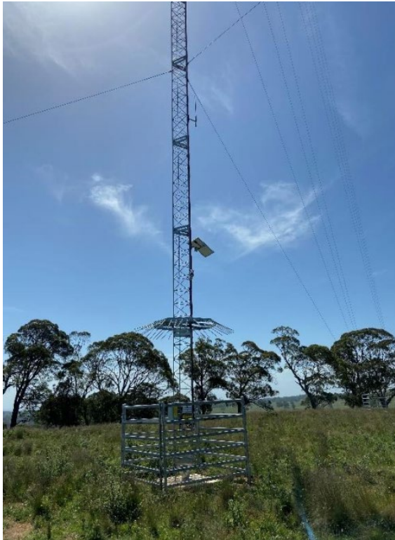
Plate 2: Meteorological mast base (105m), logger and fencing enclosure
