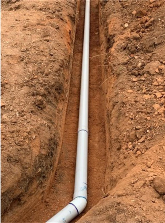
Figure 3 - Sanitary drainage installation
