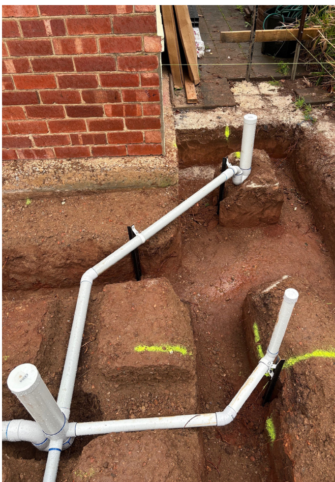
Figure 2 - Star picket pipe supports installation
