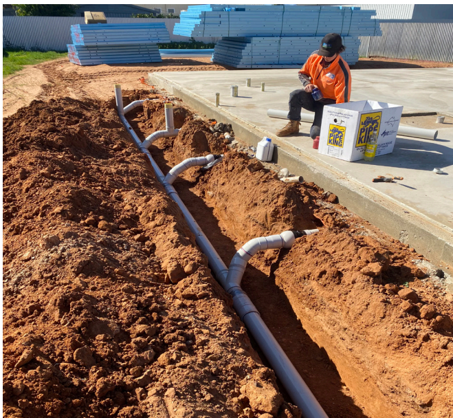
Figure 1 - Base of trench installation
